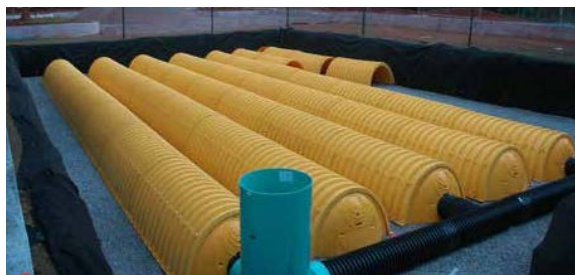
Underground cisterns collect rainwater for reuse or infiltration
