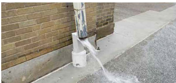
Existing downspout disconnected to drain to permeable concrete
