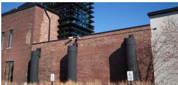
Vertical cisterns collect rainwater for re-use in irrigation
