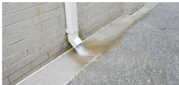
New downspout designed to drain onto permeable concrete
