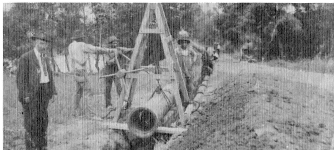
Laying the pipeline
